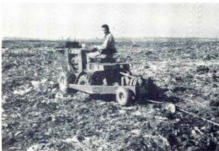
(Left, above) Technician laying ground radials—150 for each of the three towers. (Left) Extending the radials required use of a Ditch Witch. (Above) Allis-Chalmers 200-kW Diesel power generator gets a test startup. Generator will start and cut over automatically in power failures.
